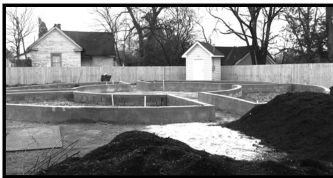
Construction Underway at the New Community Garden
